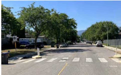
Example of a mid-block curb extensions using TCCs.
