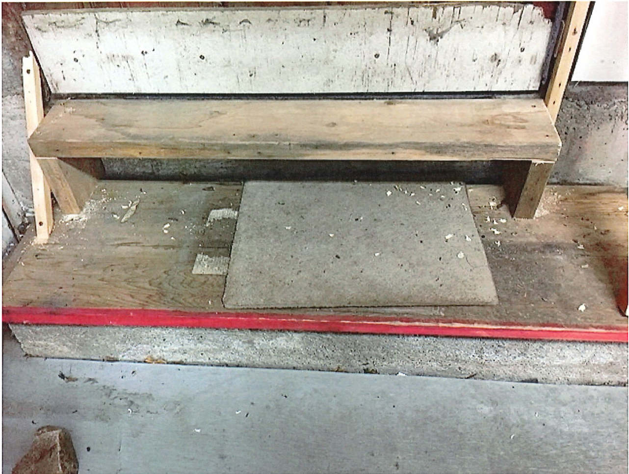
The non-compliant stairs to the Thrift store's back door, 2020.
