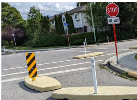
Example of curb radius reduction using TCCs.
