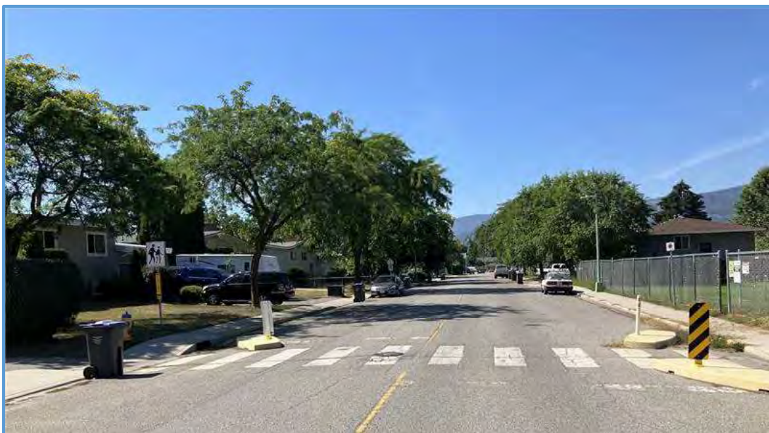
Figure 6: Midblock Crosswalk with Temporary Traffic Calming Curbs
