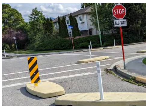
Example of curb radius reduction using TCCs.
