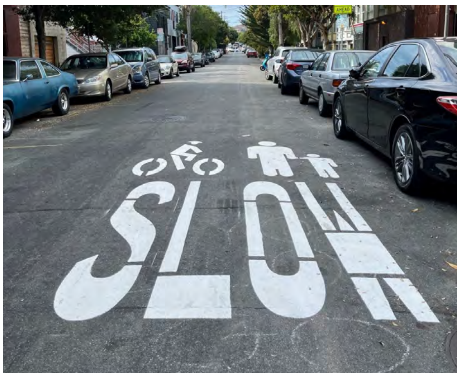
Figure 26: Example of pavement markings that help communicate roadway conditions and encourage slow vehicle speeds. Image credit: SFMTA
