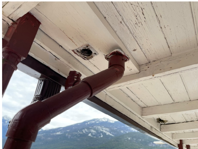
Downspout not connected to the lead scupper
