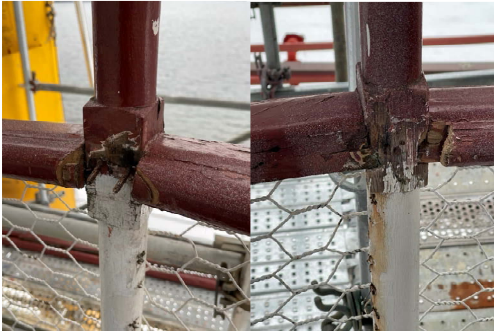
Examples of rotten spindles to railing connections
