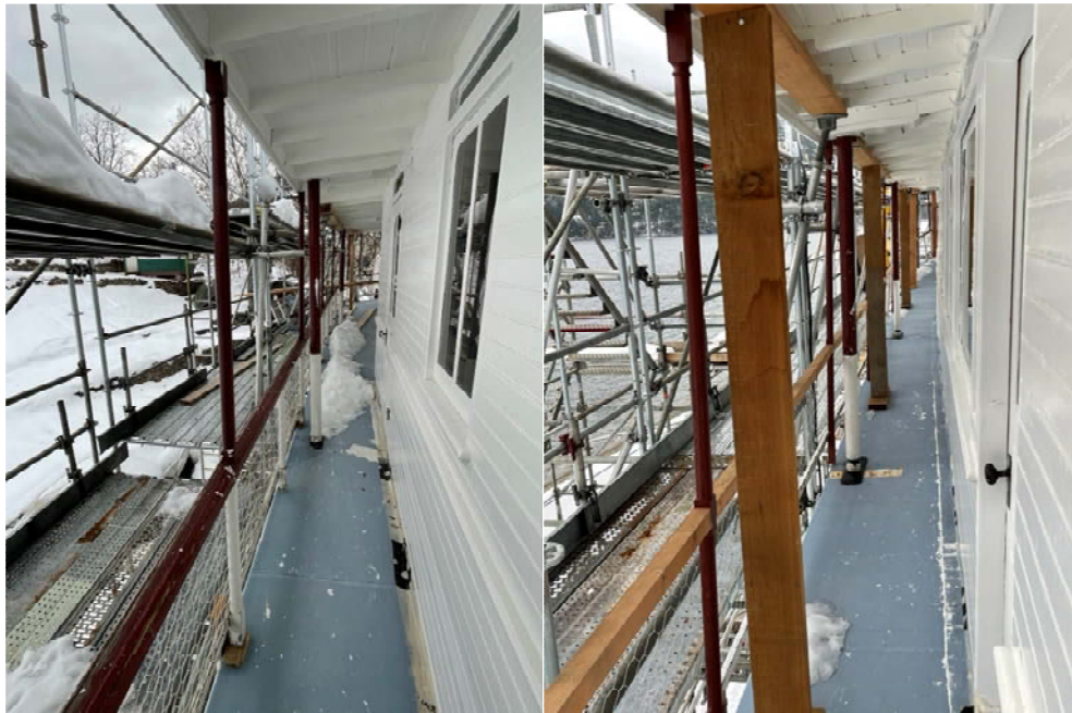
Example of the full length spindle supports and temporary supports
