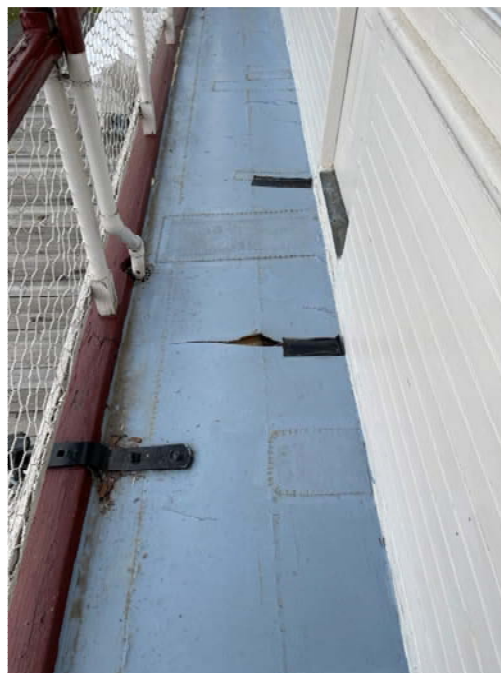
Downspout not connected to open drain lead scupper. The condition of the canvas is prior to its replacement
