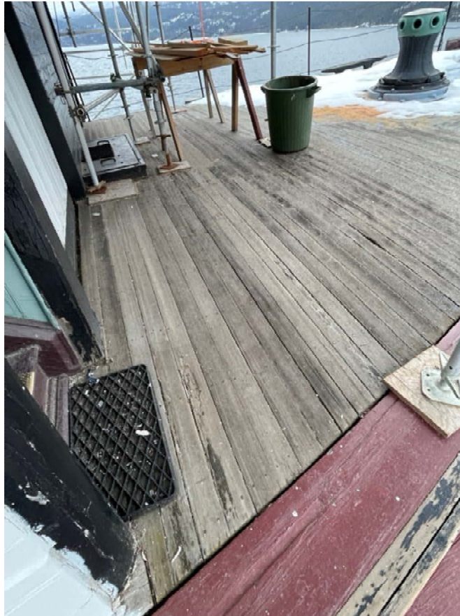
Foredeck tongue and groove construction
