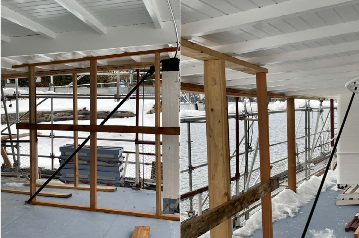
Aft deck temporary starboard and port deck supports
